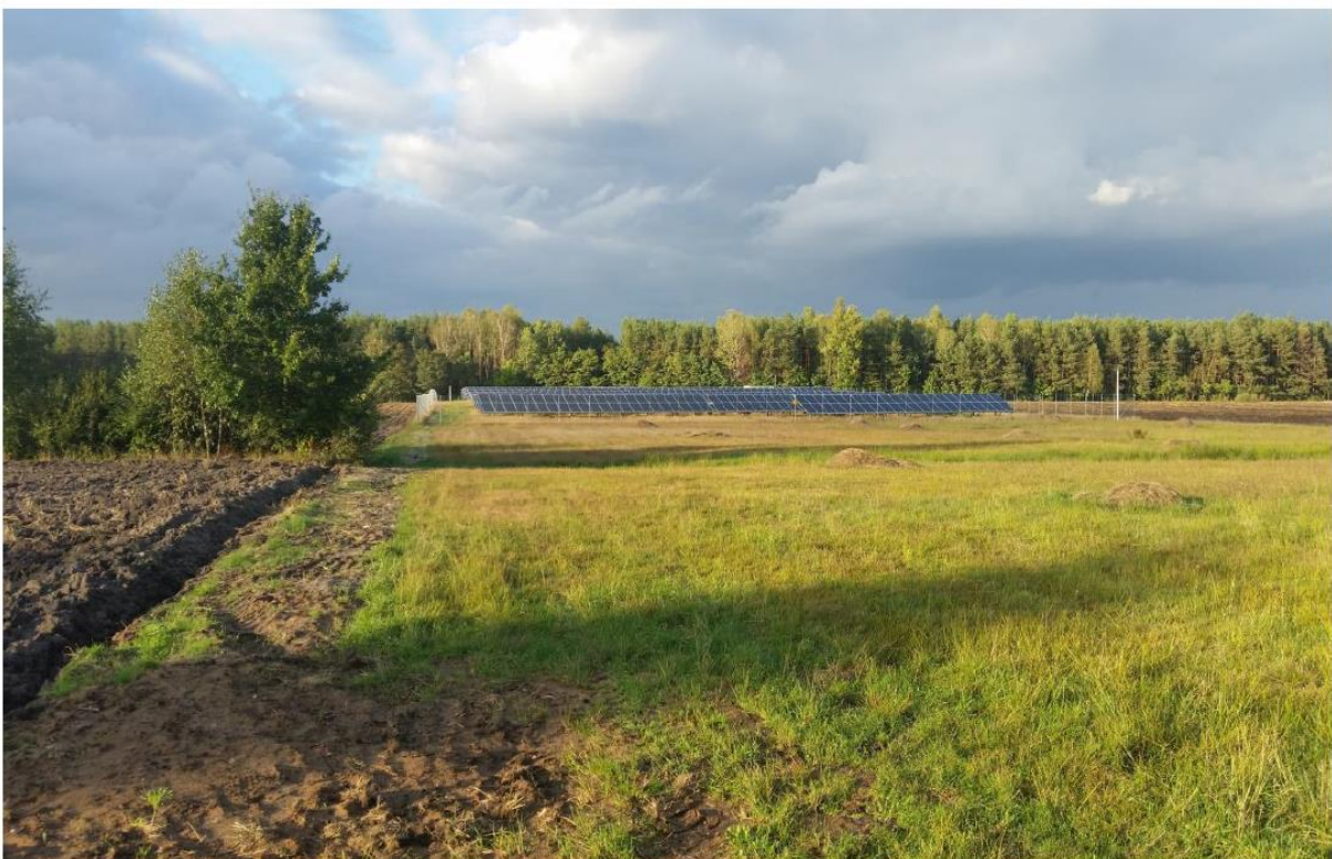
Z-5.2 Photographs of an example photovoltaic system (solar power station) built in Poland.
